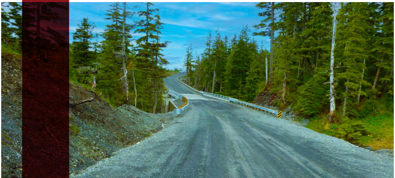
Whitshed road bridge. Cordova, Alaska.
